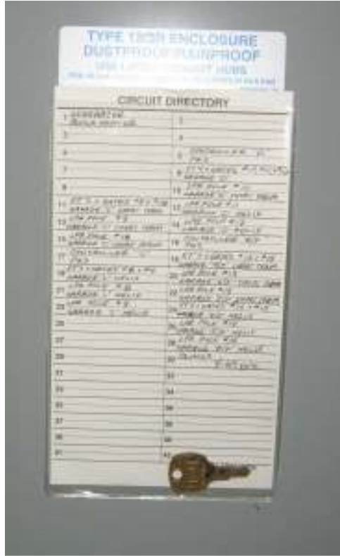
Panel EP-2B Circuit Directory Card
